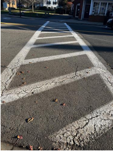
Street level view of existing Concord Center Crosswalk
