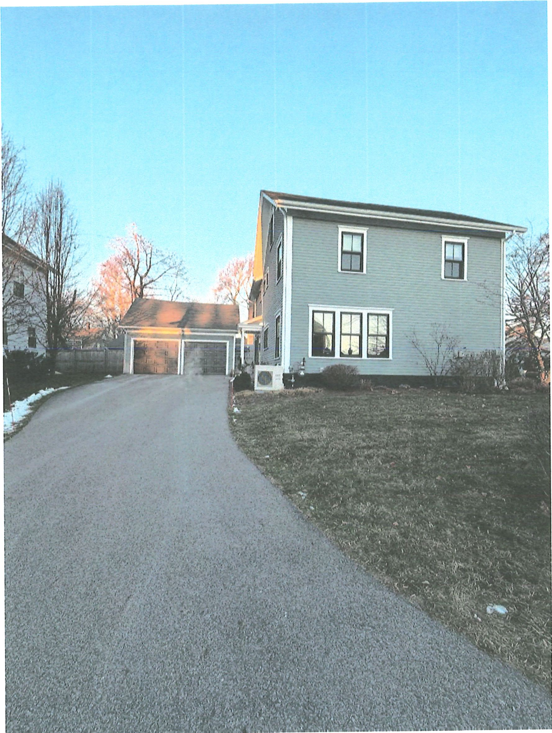
VIEW FROM HUBBARD STREET
