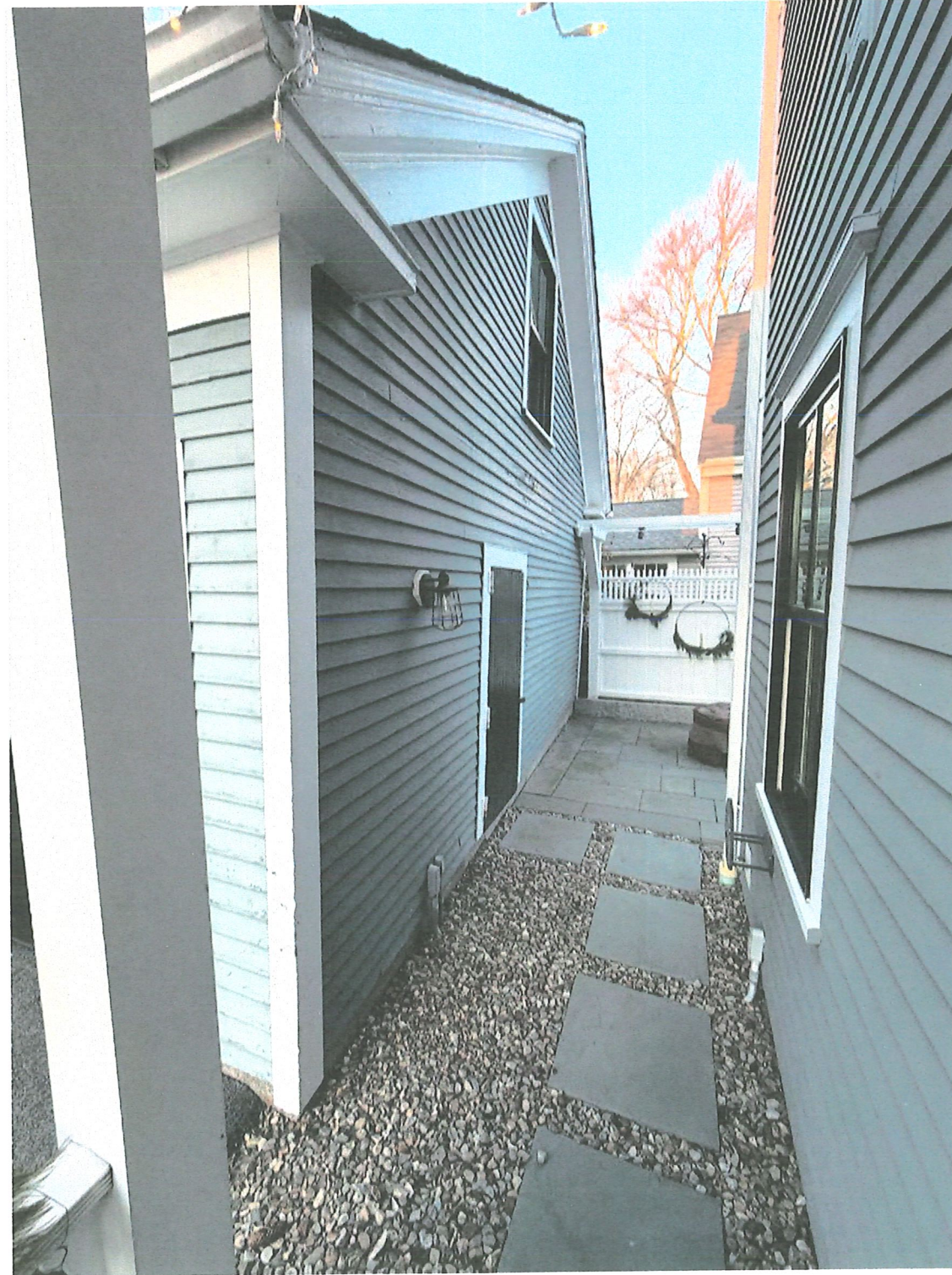
VIEW TO AISLE BETWEEN GARAGE AND PRINCIPAL DWELLING
