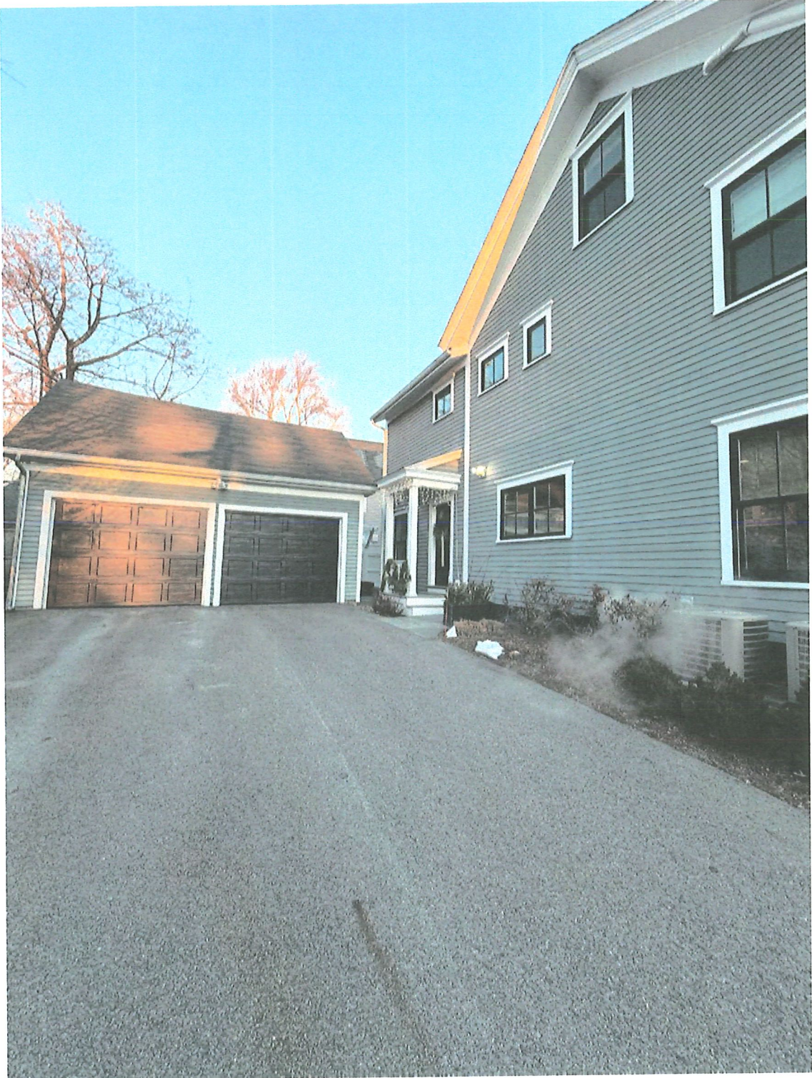
VIEW FROM HUBBARD STREET
