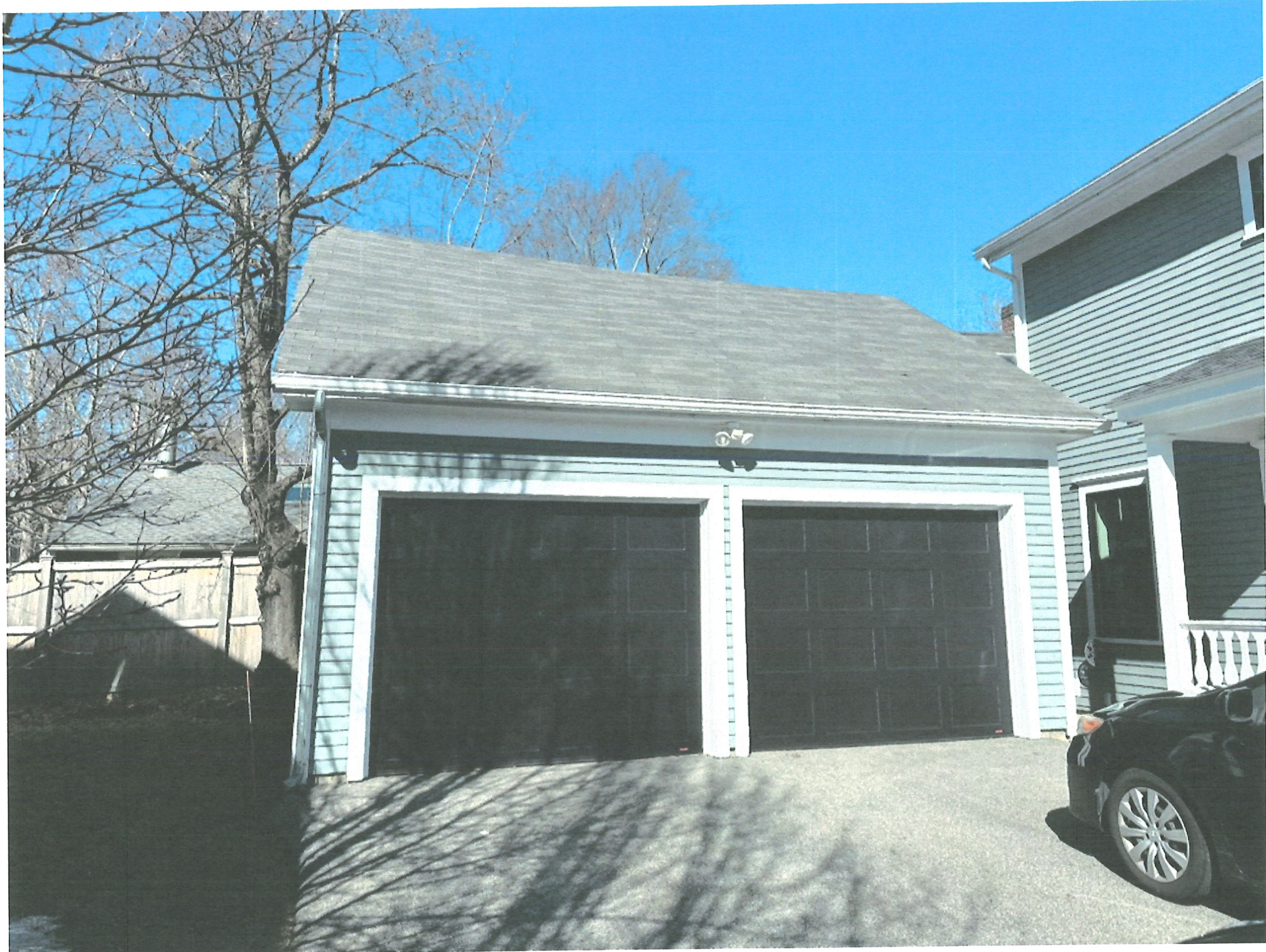
VIEW TO GARAGE
