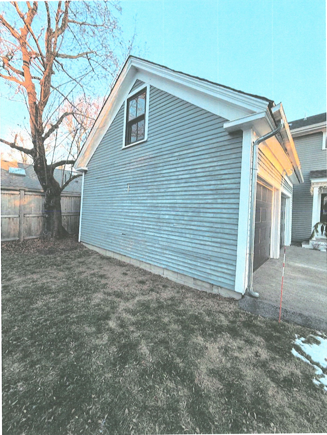
VIEW OF SIDE FACING ELEVATION
