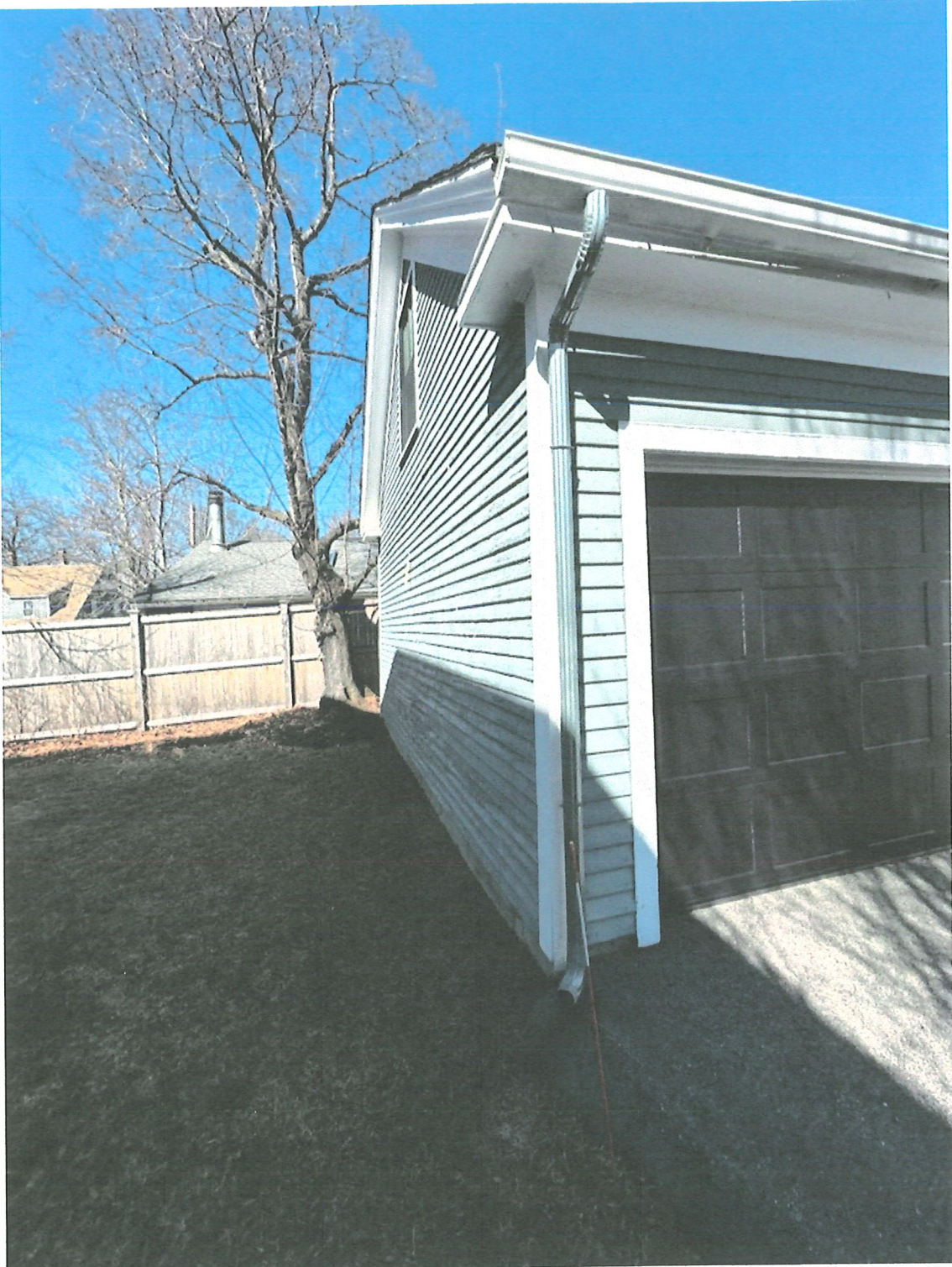
VIEW OF SIDE FACING ELEVATION
