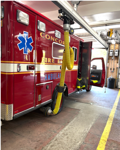
West Concord Fire Station, Ceiling height too low for many trucks
