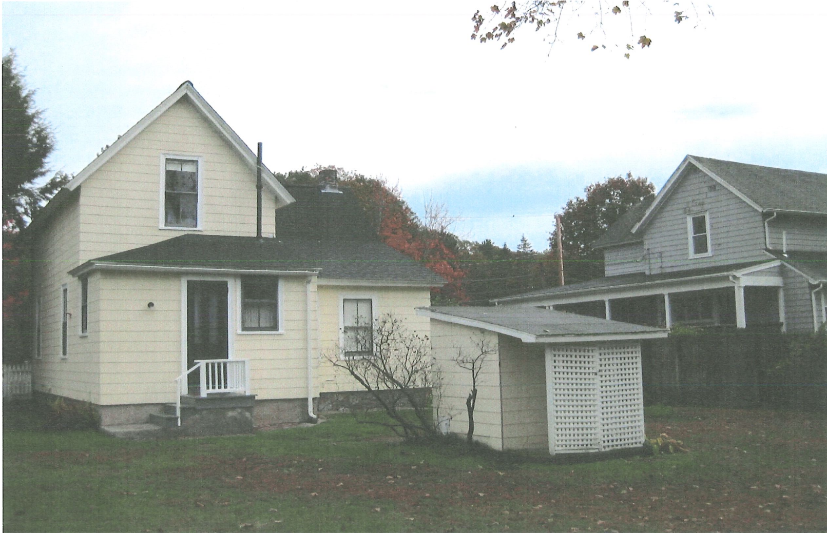
62 Crest Street - Rear View with accessory yard storage shed (To be removed.)
