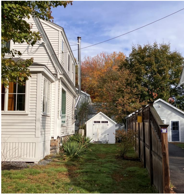
36 Pond St. – side of house of house and shed
