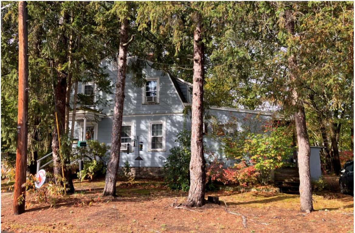
31 Pond St., Directly Across Street Neighbor to West
