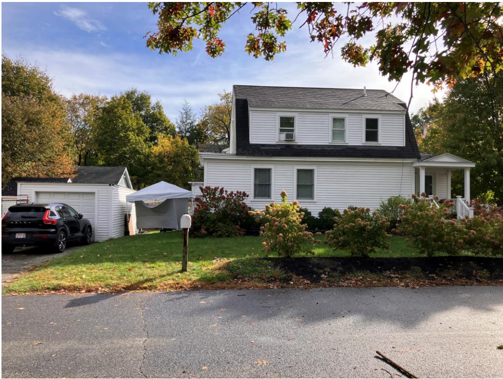
36 Pond St. view from Pond Street
