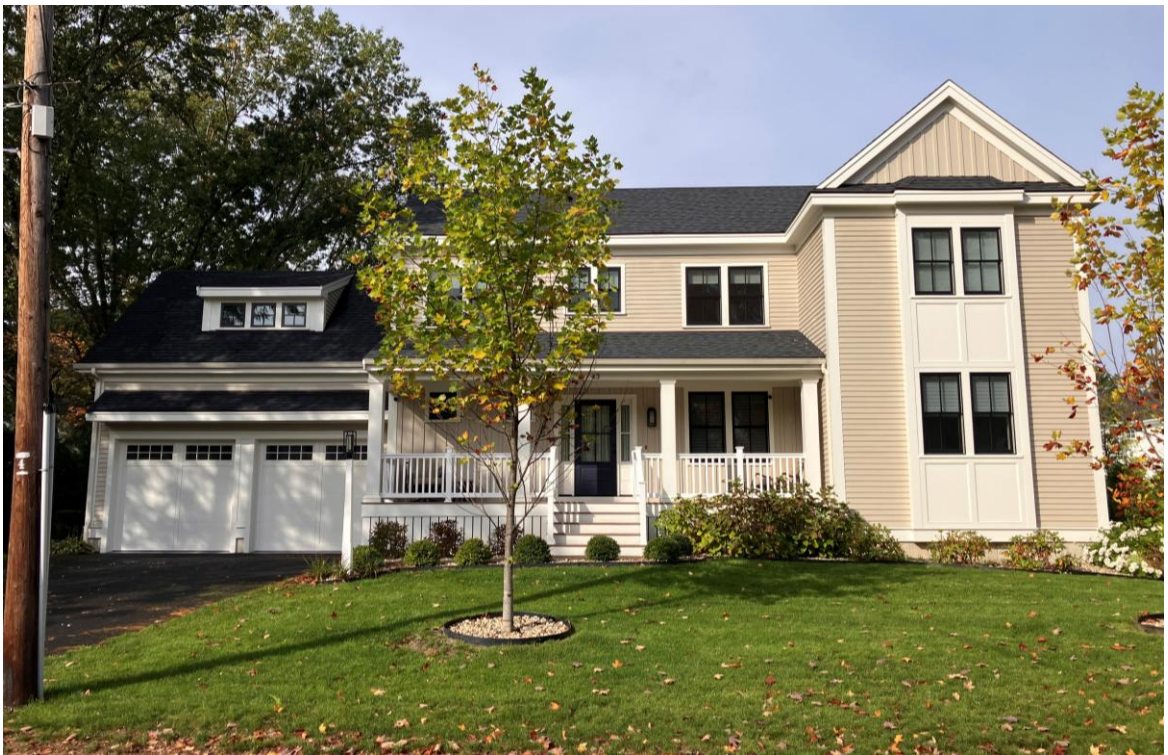
43 Pond St., Directly Across Street Neighbor to West
