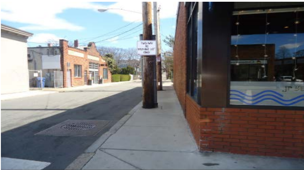
Figure 1: An example of a potential variance needed because of a limited ROW width.
