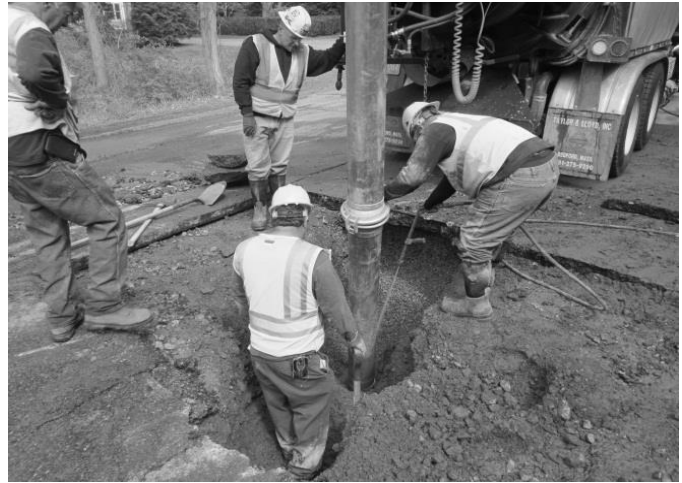
Water Main Repair on Cambridge Turnpike
