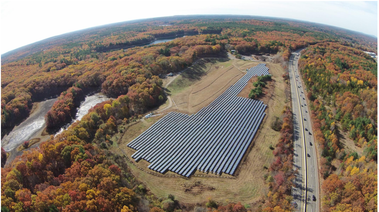
Aerial view of the solar array located at the closed and capped landfill on Route 126 and Route 2 looking west (credit: Steven Ng, member of the Concord Select Board).
