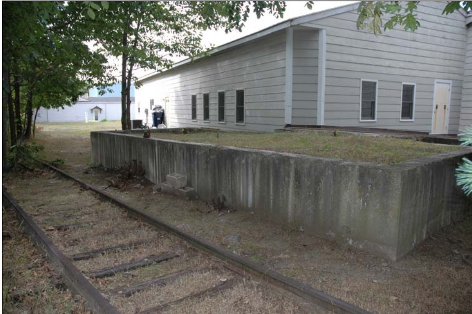
Photo 20. Resource 20, Warehouse foundation, looking southwest.
