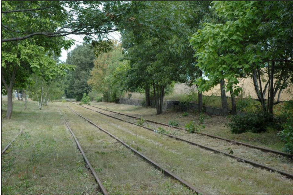
Photo 11. Resource 11, Retaining wall and multi-track yard, looking northeast towards Middlesex Junction.
