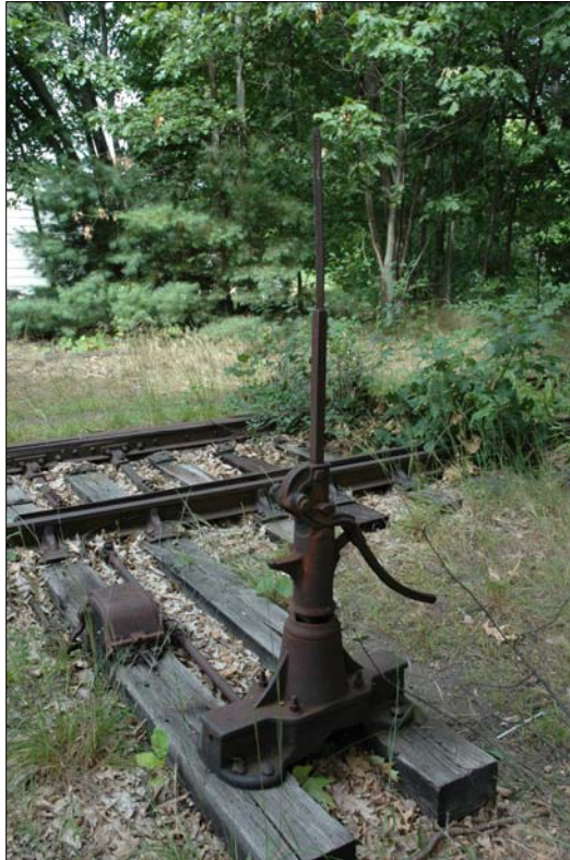
Photo 18. Resource 18, Switch, looking west.
