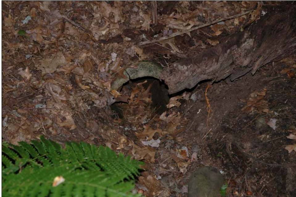
Photo 47b. Resource 48, Farm crossing culvert detail, looking south.
