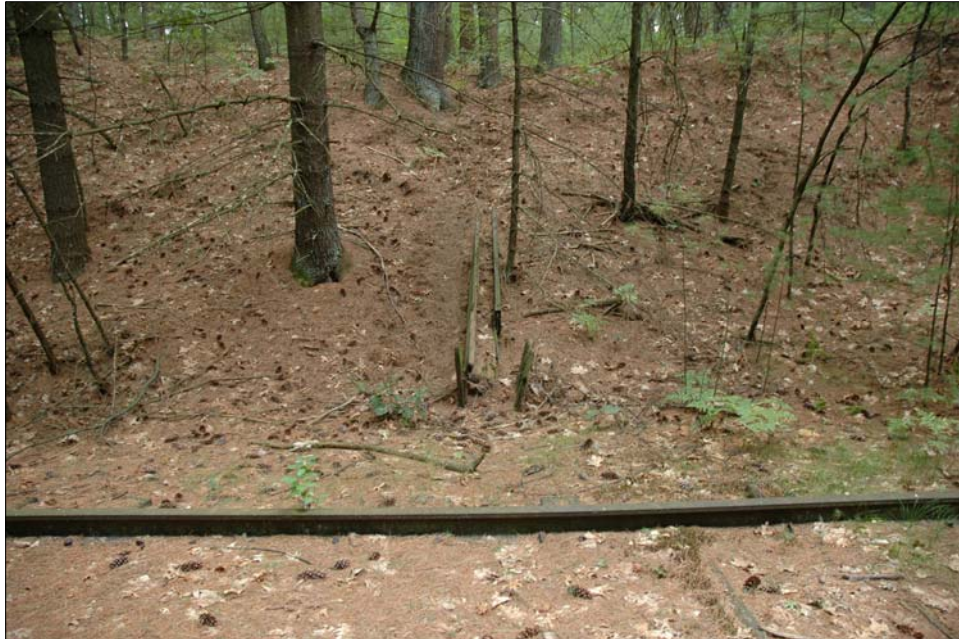
Photo 43. Resource 44, Trough or conduit, looking west.
