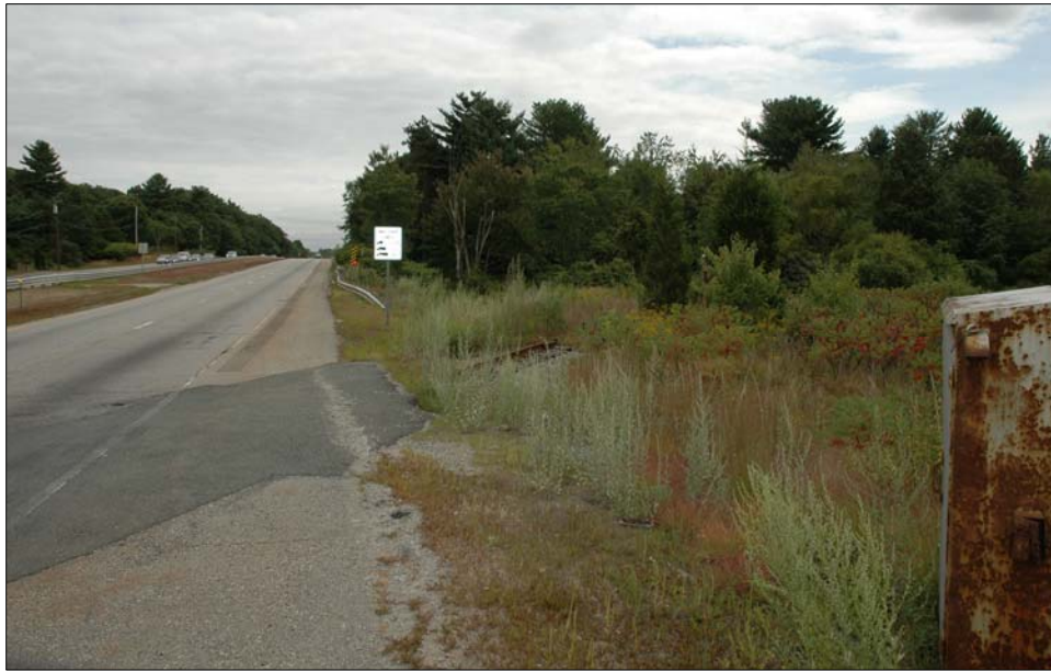
Photo 1. Resource 1, Beginning of extant rail and ties, looking southeast.
