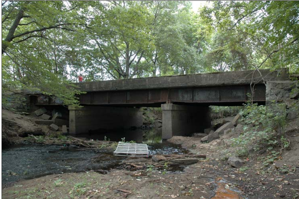
Photo 16b. Resource 16, Southerly Nashoba Brook Bridge, looking southwest.
