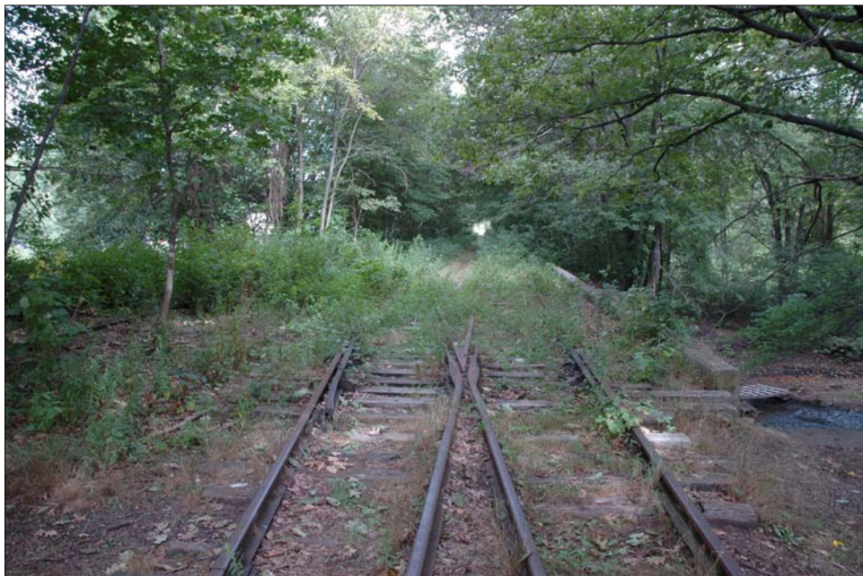
Photo 16a. Resource 16, Southerly Nashoba Brook Bridge, looking north.
