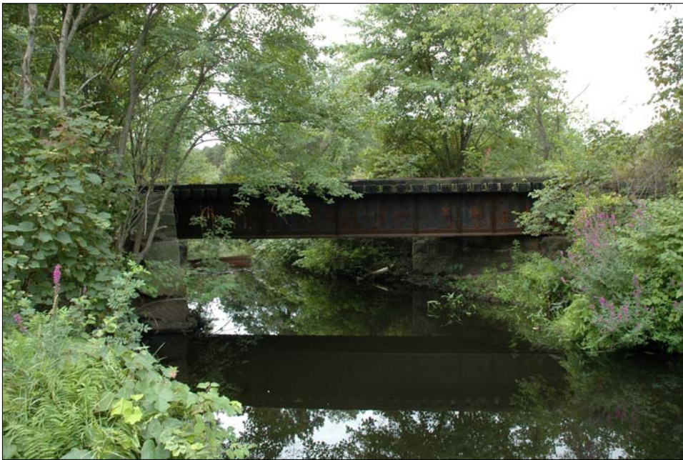
Photo 4b. Resource 4, Northerly Nashoba Brook Bridge, looking south.
