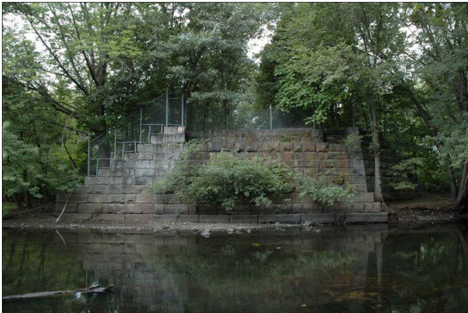
Photo 29a. Resource 29, Assabet River Bridge, north abutment, looking north.
