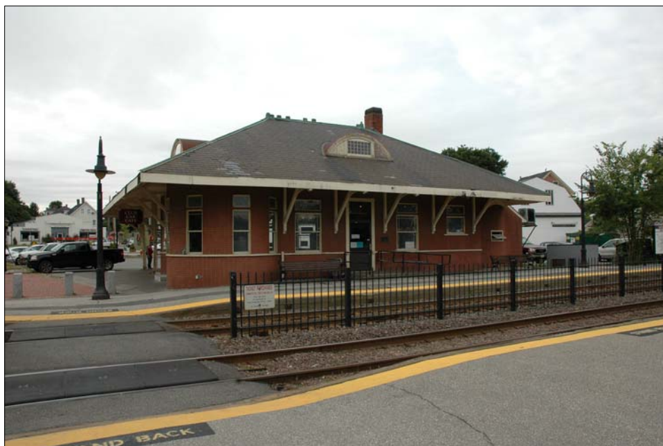
Photo 23. Resource 23, Union Station, looking south.
