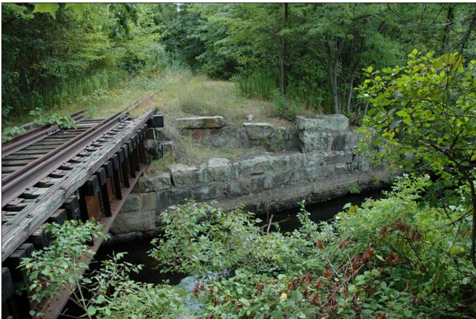
Photo 4c. Resource 4, Northerly Nashoba Brook Bridge, detail of east abutment showing seat for second bridge span, looking southeast.
