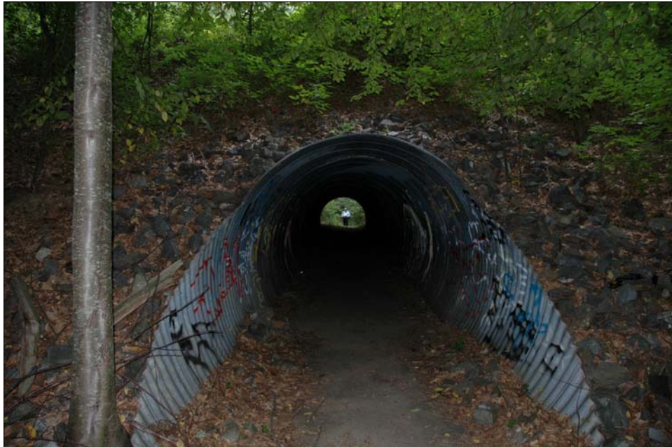
Photo 48. Culvert on railroad right-of-way below Powder Mill Road, looking north.
