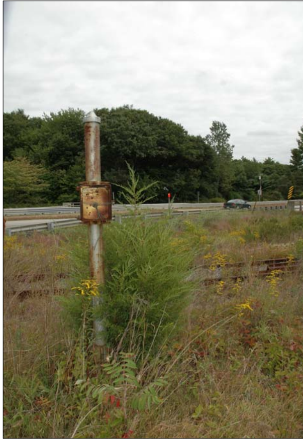
Photo 3. Resource 3, Relay box on pole, looking east.
