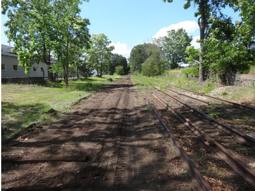
LOCATION WHERE RAIL HAS BEEN REMOVED
