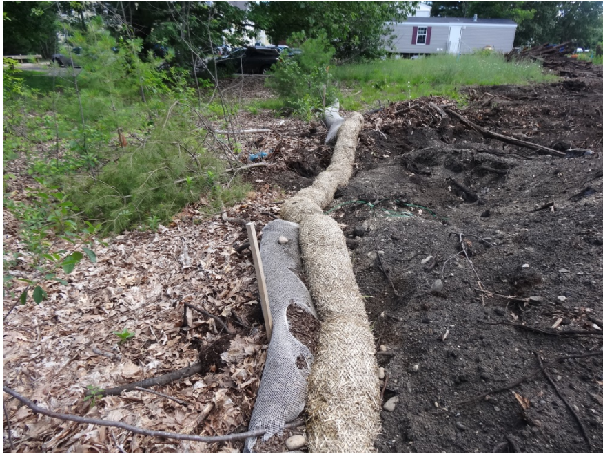
DAMAGED EC HAS BEEN REPAIRED
